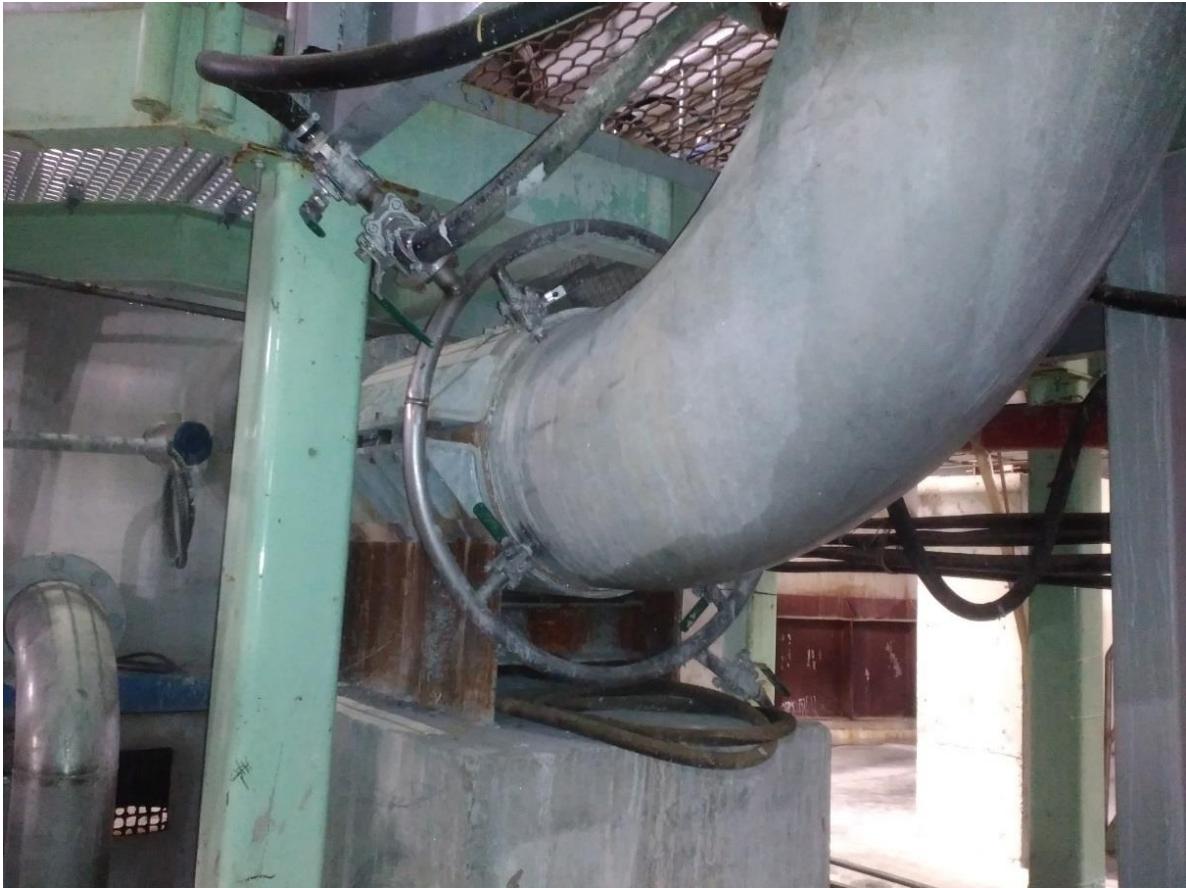
Picture 1 – Chemical feed system for retention on PM 7
